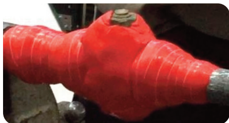
Corroded valve wrapped in LLFA Smooth
