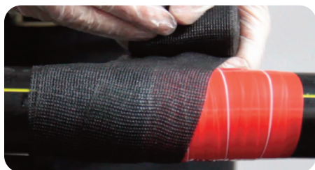
LLFA Garde reinforced squeeze-off
