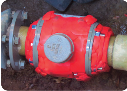
Filled uneven surfaces with LLFA Smooth
