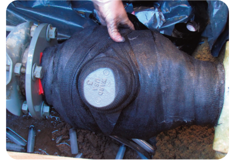
Finished with a layer of LLFA Garde
