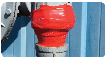
A leaking riser stopped with LLFA Tape
